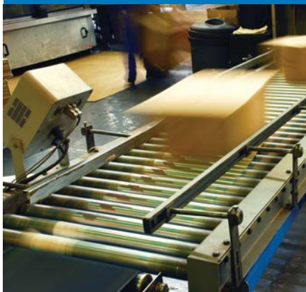
Pneumatic cylinder replacement, product diverter for conveying line.
